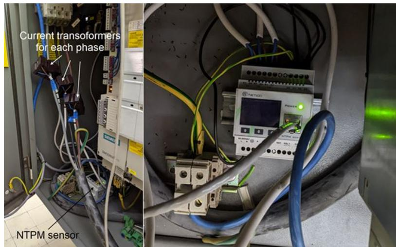
**Fig. 2** NTPM smart sensor aimed for measuring electric magnitudes
