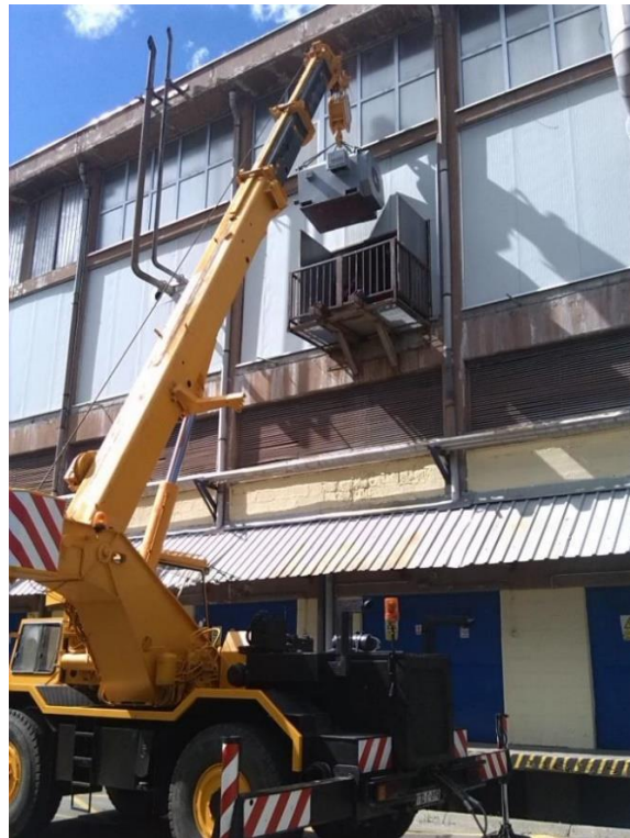
Fig. 6 Logistics of maintenance activities
